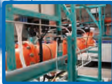
Rampe Metano (Taiwan)
