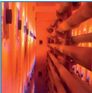
CONTROLE DE TEMPERATURE
