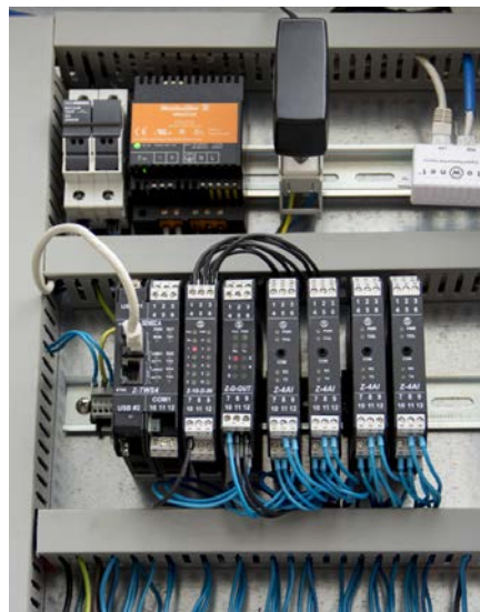
Peripheral unit panel detail
